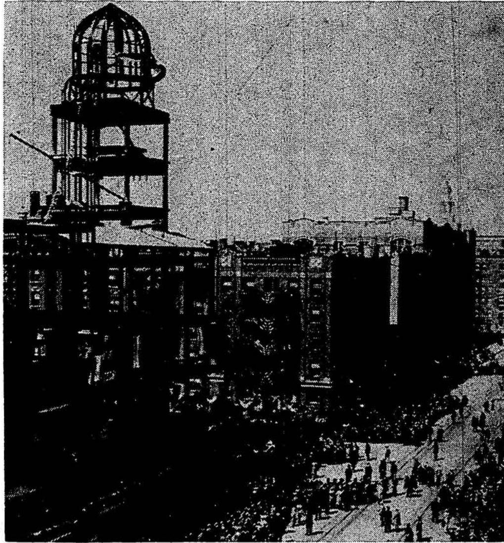
A BUILDING GOES UP: The present site of Yeshiva had not yet been completed when the dedication ceremonies took place, witnessed by an overflow crowd.
