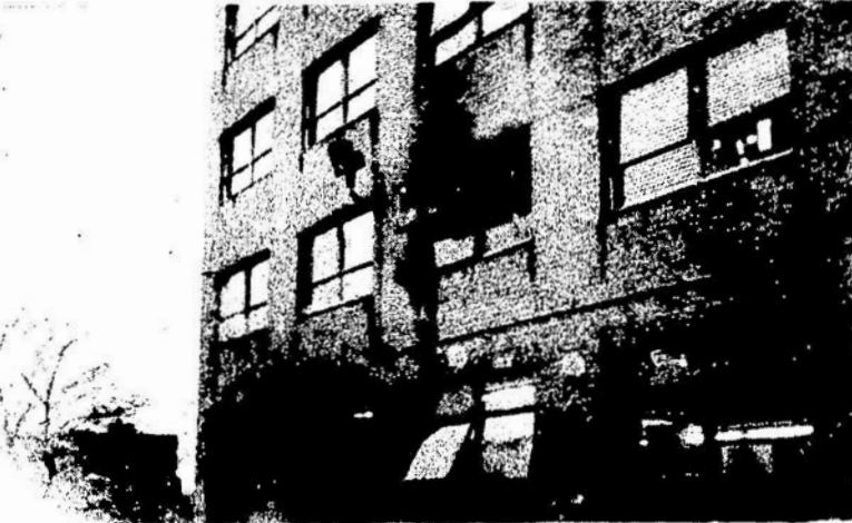
Rubin Hall damaged by fire
