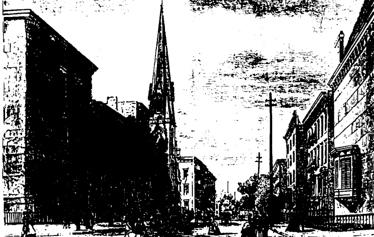
Lexington Avenue and 36th St., looking south
