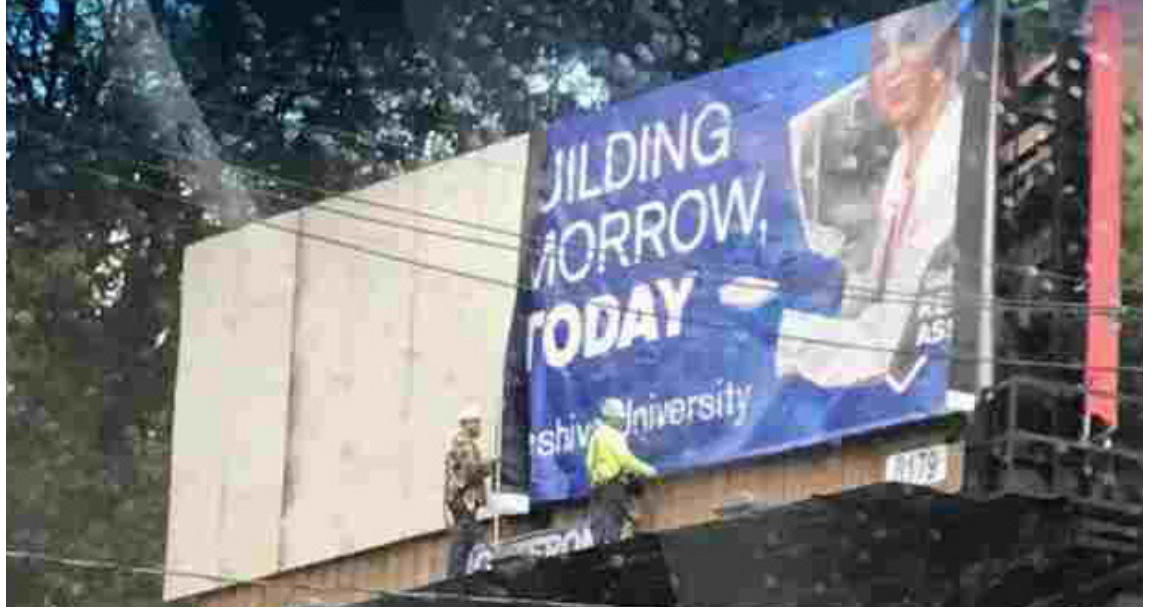
Yeshiva University Route 4 Billboard Being Installed
