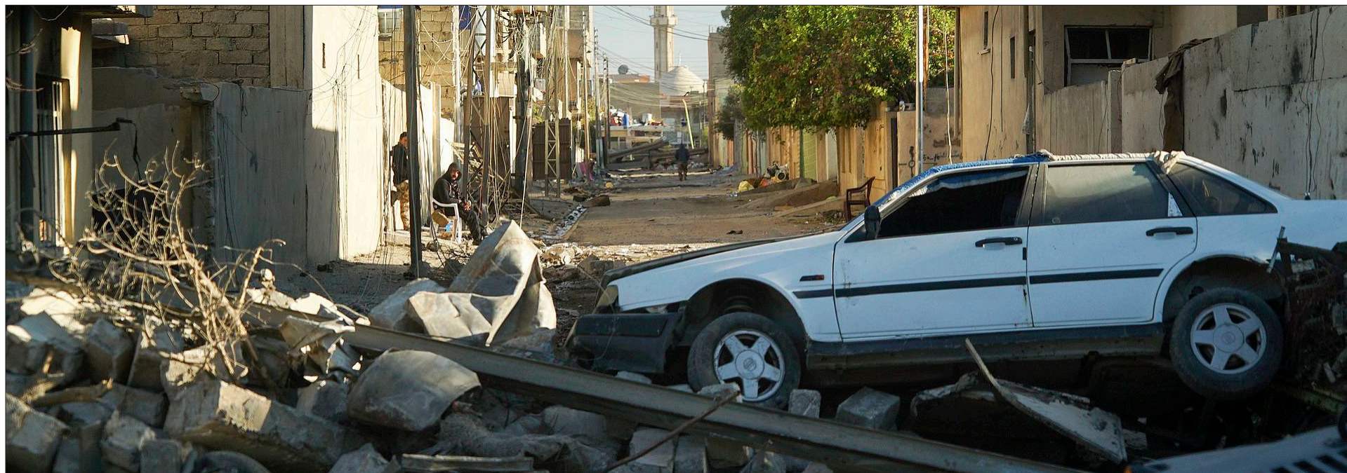
Ruins of the blast site
