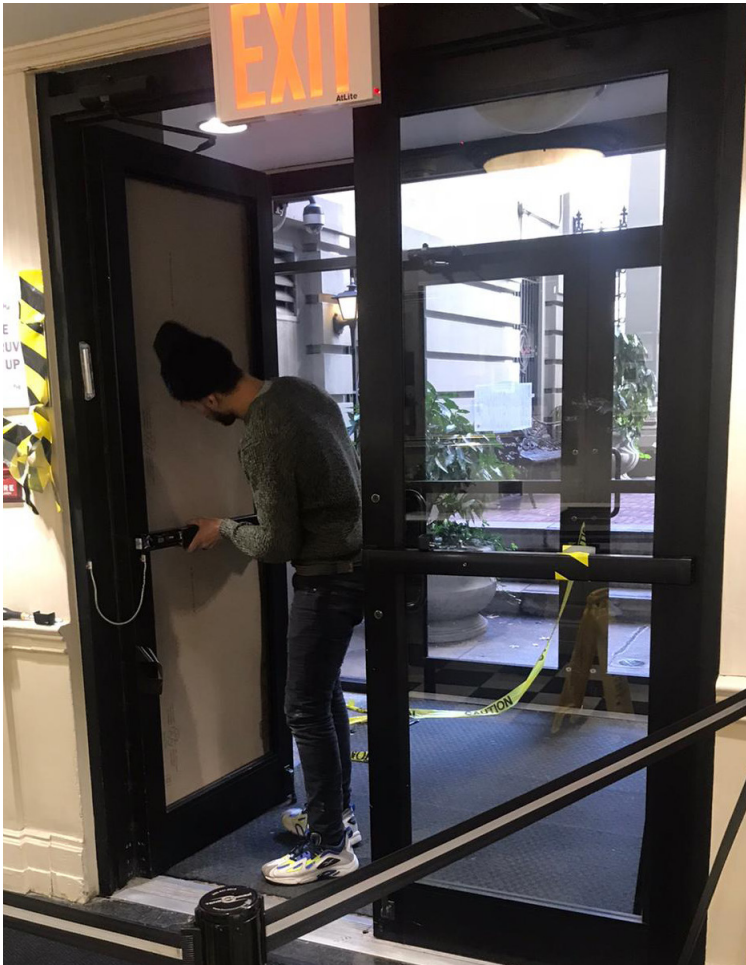
The front door was repaired on Friday.
