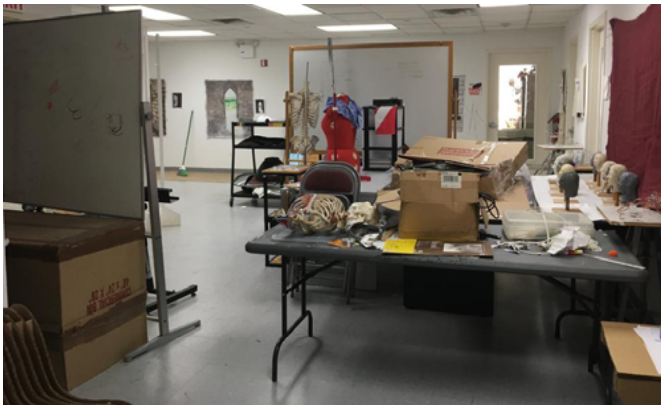
The state of the art floor during renovations
