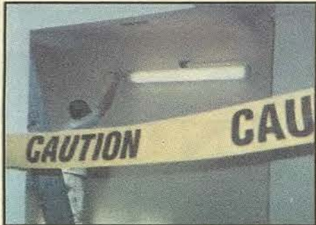
Workers hurry to finish staircase for opening on Sunday
