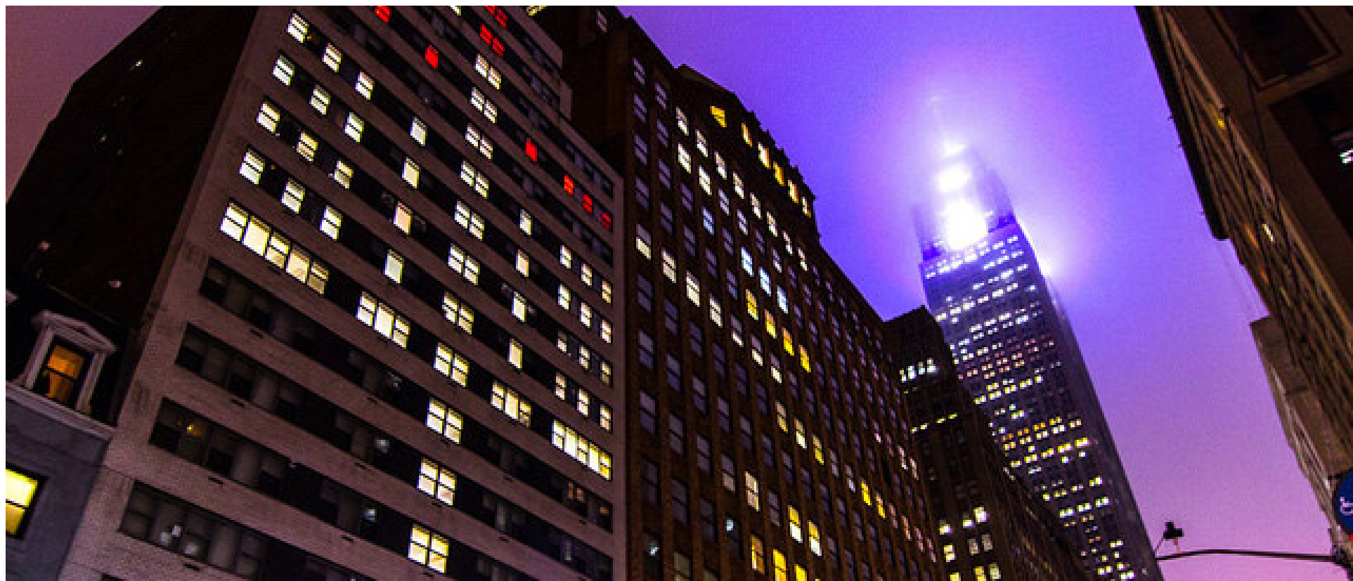
Brookdale Residence Hall
