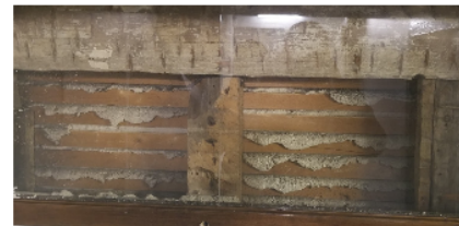
Figure 5: The interior of the walls
