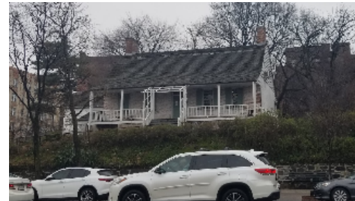
Figure 1: The house sits high above the street
