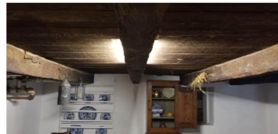
Figure 8: The beams in the basement
