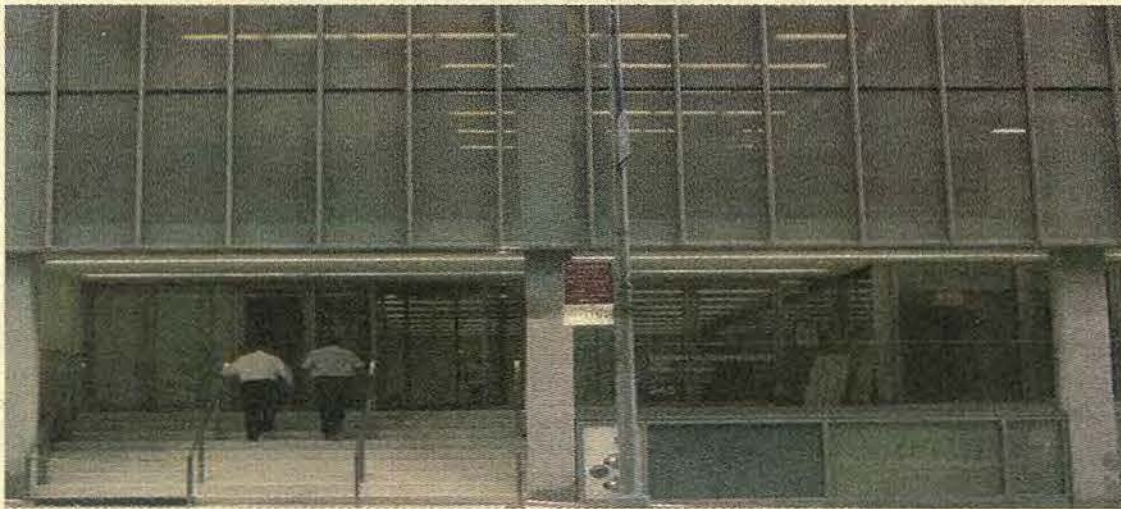
New facade of 245 Lexington Avenue nears completion.
