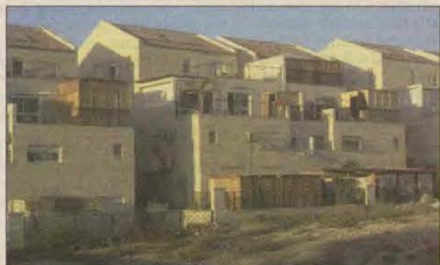
The Observer Sukkahs embellish every balcony of a Beit Shemesh apartment building.
