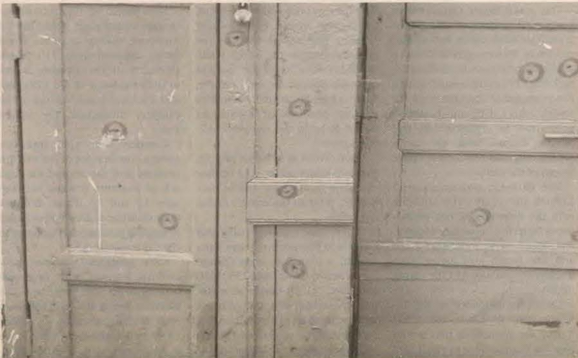
Bullet holes circled in red on the door of the Chabad Narriman House
