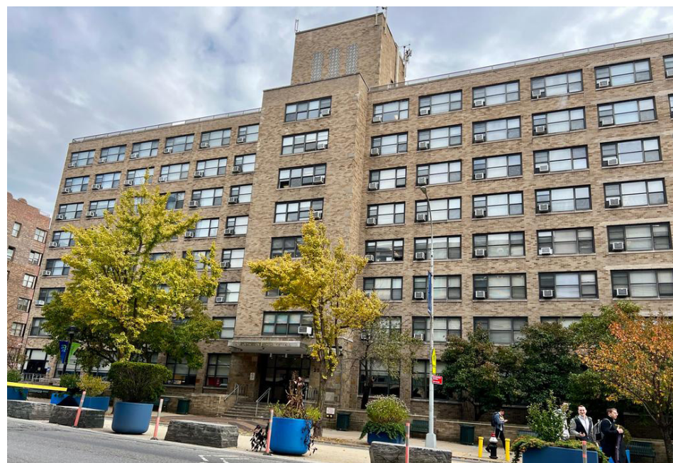
The ground floor of Morgenstern Residence Hall is receiving a redesign with a new Sephardic Beit Midrash and lounge area.
