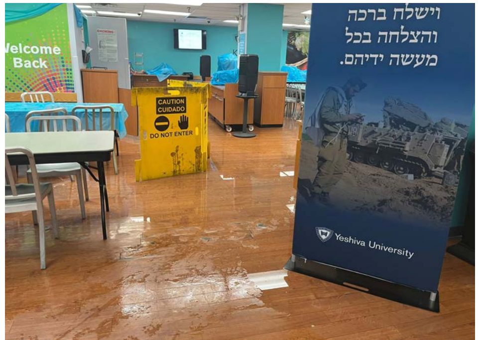
The Kushner Dining Hall was temporarily flooded Dec. 3
