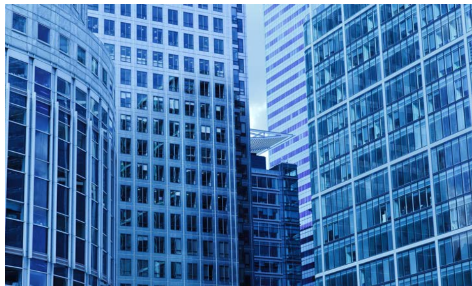
A cluster of modern office buildings through a color filter making them look a similar shade of blue/grey
